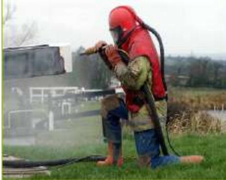
*Shot blasting using recycled glass grit on a steel lock balance beam at Devizes on the Kennet and Avon Canal*
