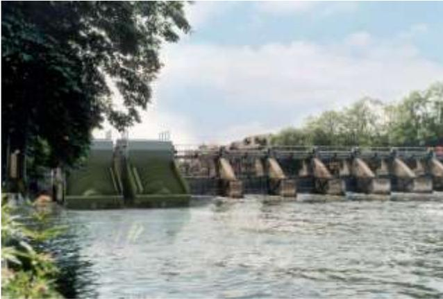
*This illustration shows how the Archimedes screws turbines would be located within Romney Weir*
